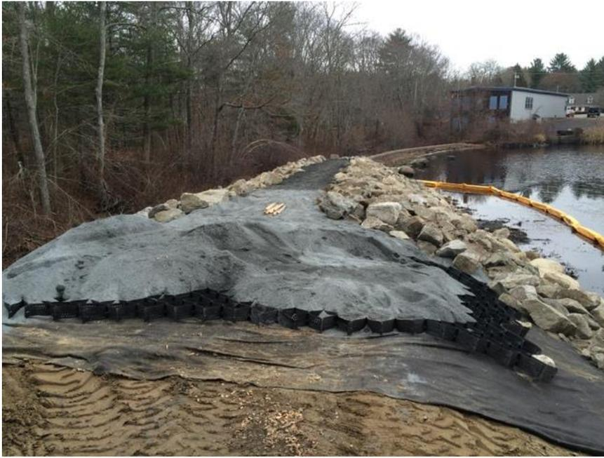
Figure 44: Factory Pond Dam, left embankment reconstruction
