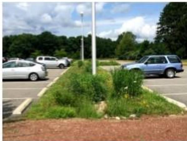
*Bioretention strips filter parking lot runoff*
