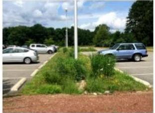
Bioretention strips filter parking lot runoff
