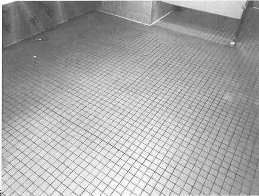
Ceramic floor tile grout/adhesive
