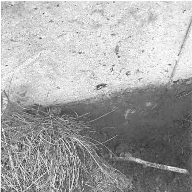
Typical view of foundation wall – no foundation mastic found
