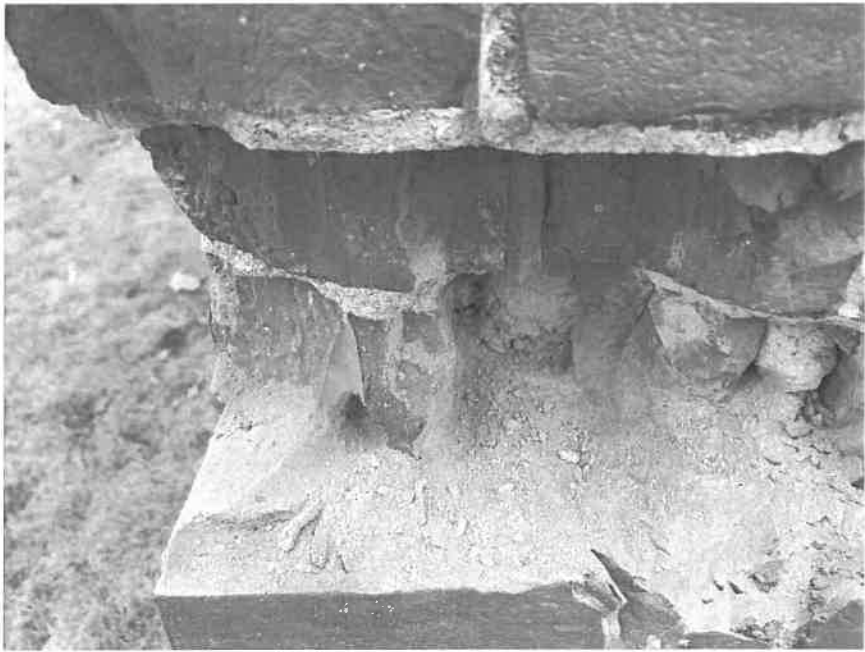
Area behind brick wall – main building
