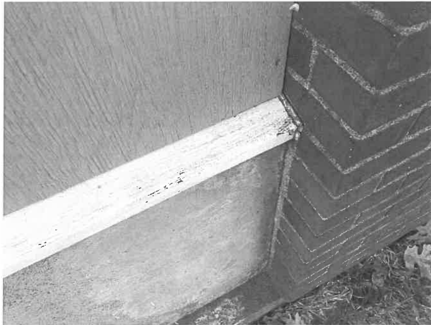
ACM exterior window caulk on Main Building and Old Extension
