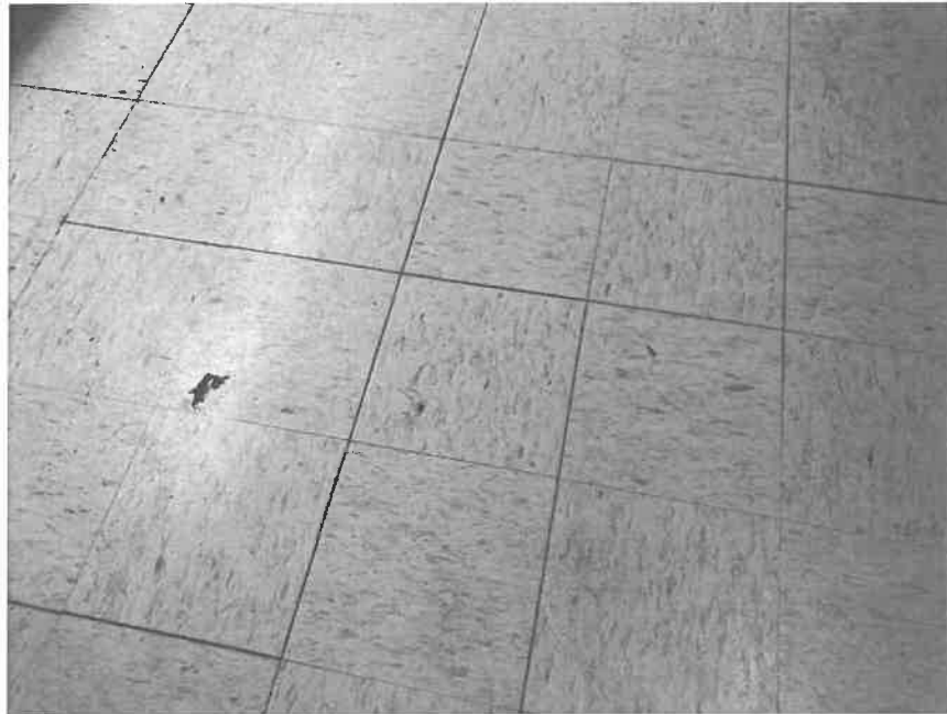
12" x 12" white with blue streak floor tile. Note – mastic is ACM.
