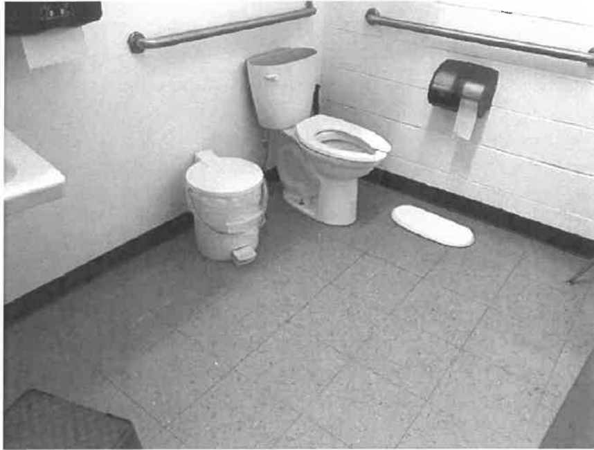
12" x 12" brown floor tile in New Extension
