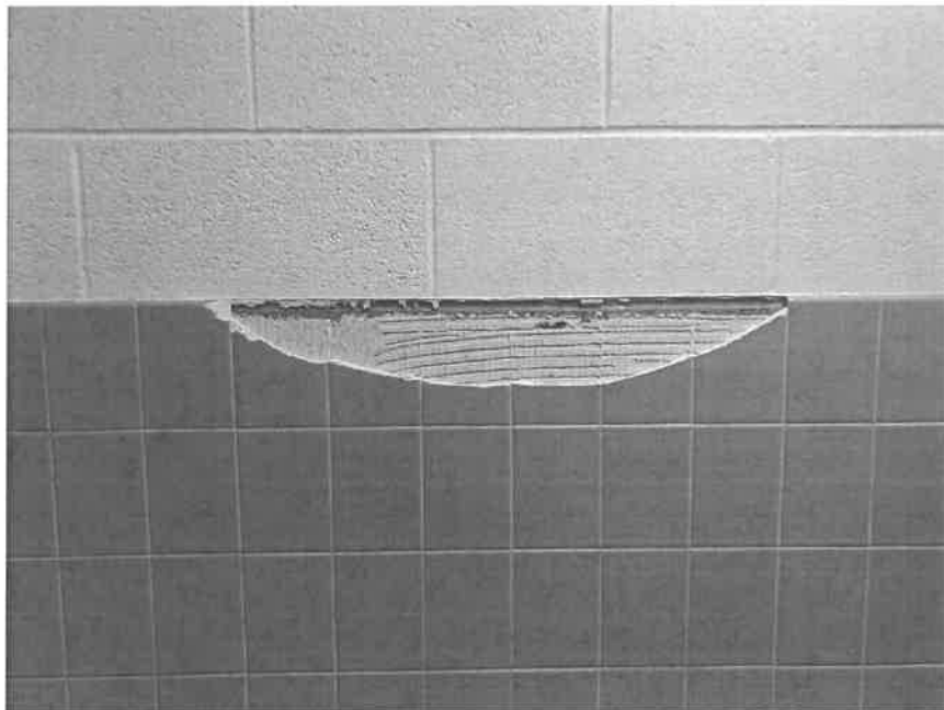
Ceramic wall tile grout/adhesive
