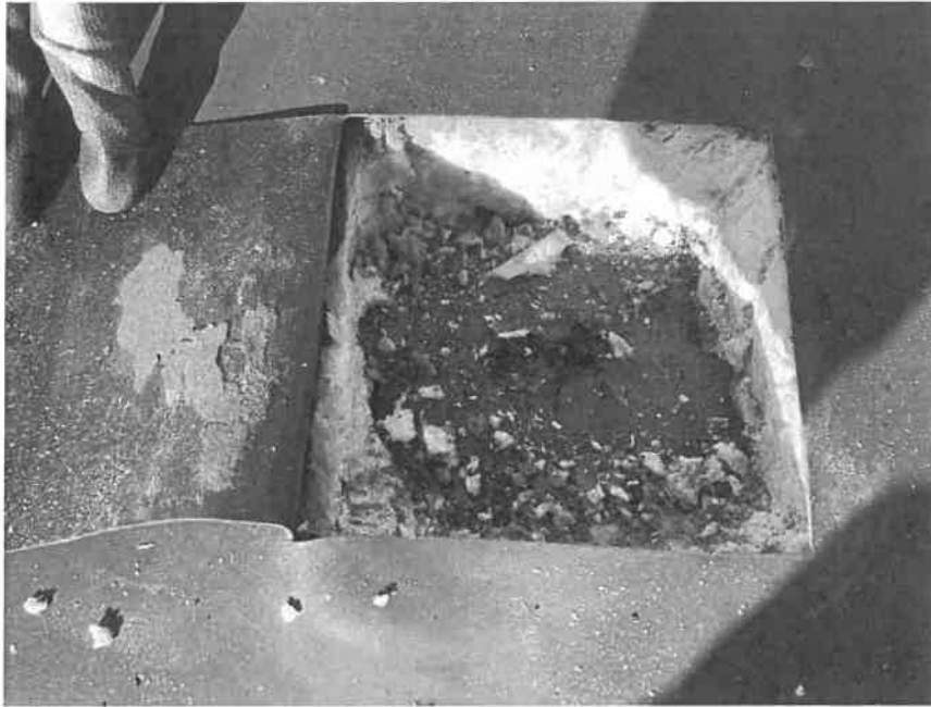
Typical roofing system at site.
