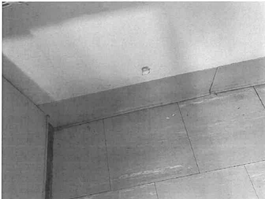
ACM cement panelboard by radiator, non ACM 6" beige cove base/adhesive
