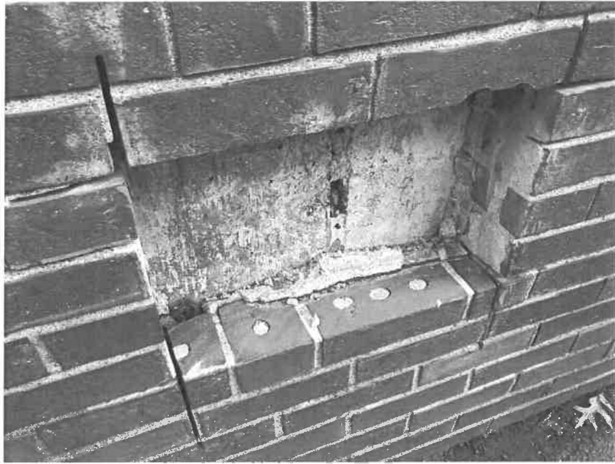
Area behind brick wall – Old Extension
