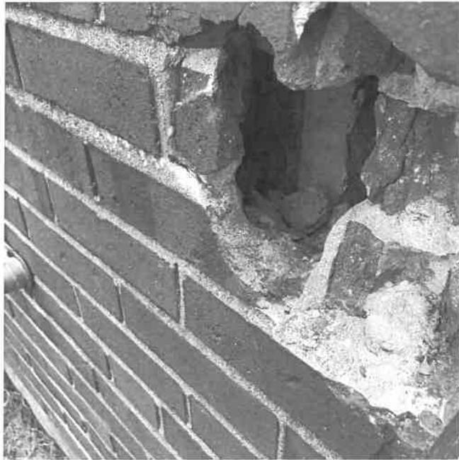
Area behind brick wall – New Extension
